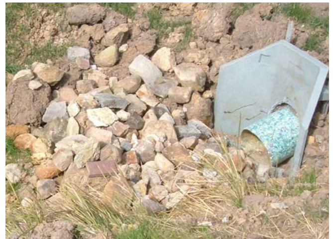
Above: Rock protects the outlet of the dam's trickle pipe. Below: A cover crop of oats greens the new embankment.
