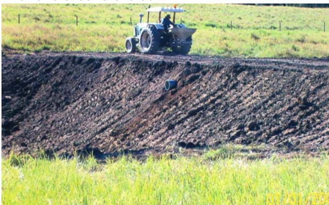
Above: Gypsum was spread on the finished embankment and dam surrounds.
